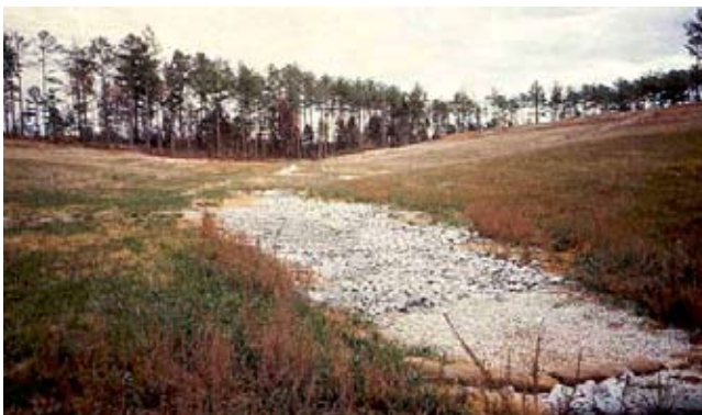
Figure TS14P-34 Reshaped gully with rock-filled concentrated flow channel, Union County, SC, 1987
