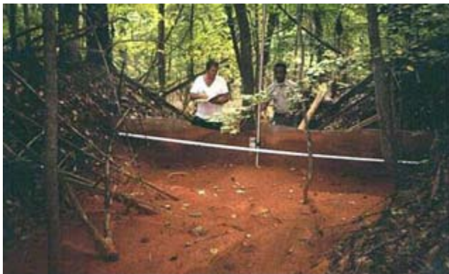
Figure TS14P-13 Erosion resulted in sediment from a small gully trapped in filter fabric fence
